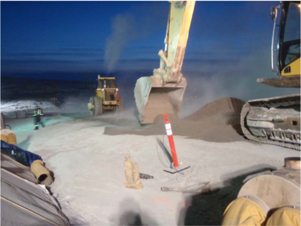
Photo 5: Excavator spreading a thinner lift towards the northeast end of the dam.
