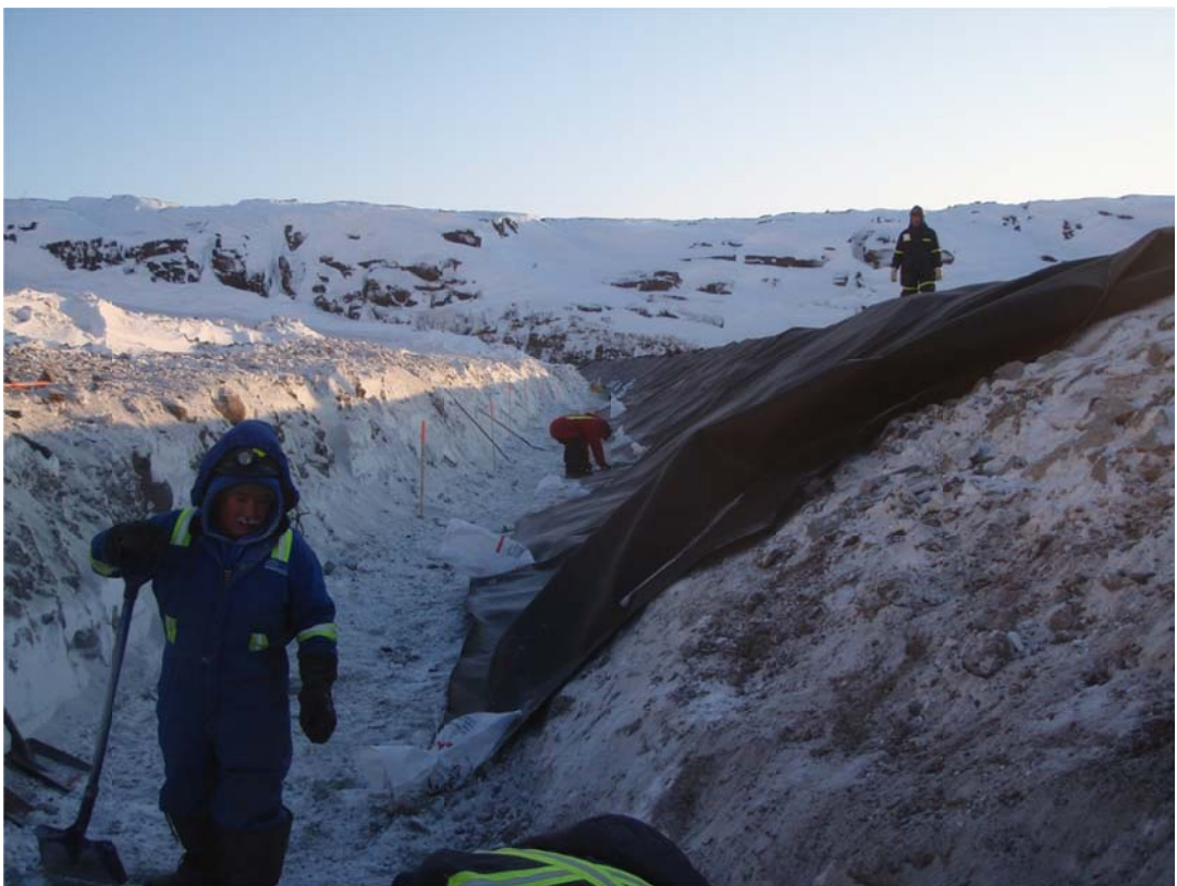
Photo 9: Foreground: Labourers cleaning snow prior to liner placement. Background: Layfield installing non-woven geotextile.
