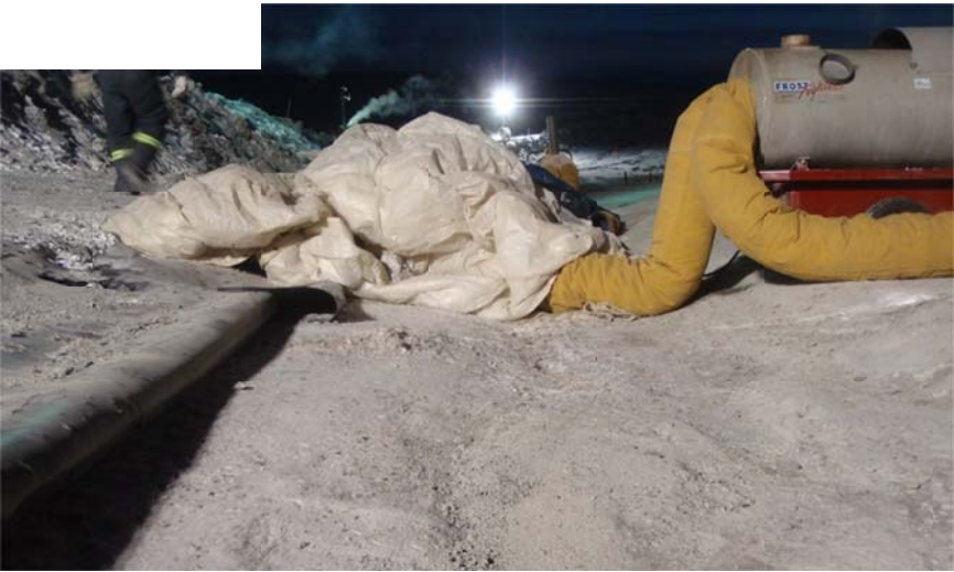
Photo 4: Hoarding tents set up on liner exposure. Fewer tents are currently being used with the same number of frost fighters.
